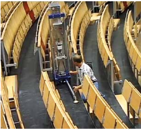
Fitting of the lower outriggers
