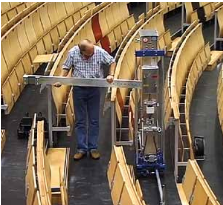
Fitting of the horizontal outriggers
